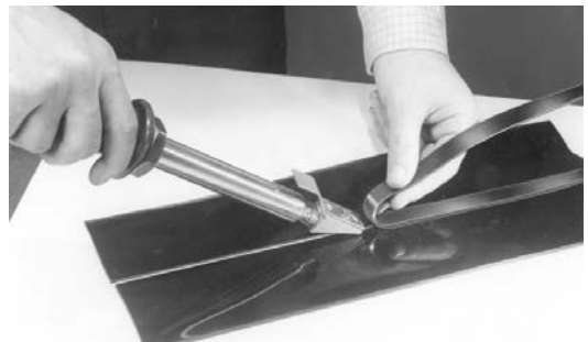
Hand Welding Flat Strip
