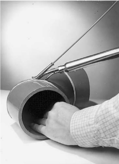
Speed Welding Pipe
