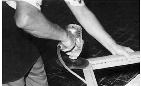
Dressing Weld with Rotary Sander
